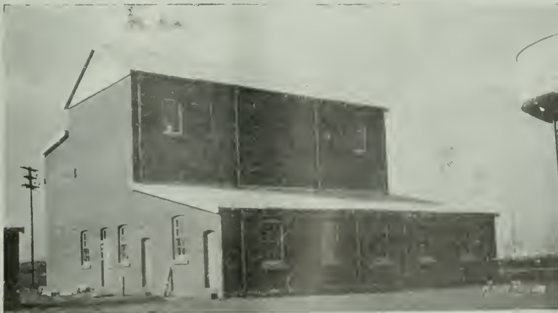
A TYPICAL TRANSFORMER HOUSE ON A RAND MINE.
